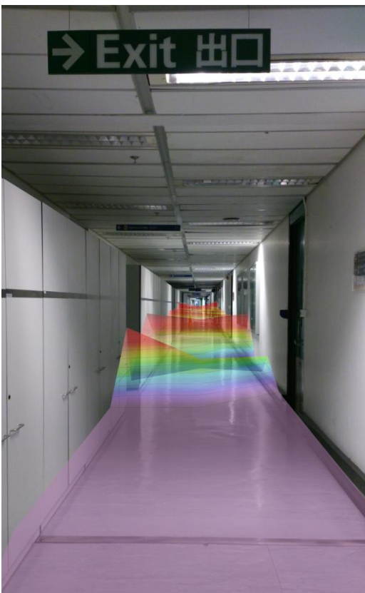
Figure 3 Front view of the 2 nd floor corridor
